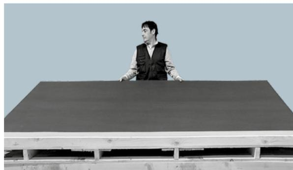
1 | 100x300 cm and 120x260 cm slabs of laminated porcelain stoneware can be lifted by one person. Lift the slab with open hands. Slowly raise the longer side so as to eliminate the suction effect, due to contact with the underlying slab, and ensure a good grip. When handling the use of gloves is recommended.
