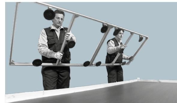
4/5 | 100x300 cm and 120x260 cm slabs of laminated porcelain stoneware can be handled by two people with the help of a special frame. Fix the frame to the slab when it is still on the pallet. Raise the frame and slab to eliminate the suction effect.
