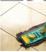
"Post-installation" cleaning helps remove residues of joint grouts, cement and lime. This operation is mandatory after installation both for glazed and unglazed tiles. Never clean tiles that are too hot (e.g. exposed to sunlight during hot summer months) since the reaction of aggressive chemicals may become harsher. In the summer, proceed with the operation during the coolest period of the day.
