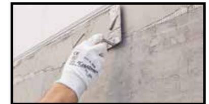
Position the profile and embed the mesh
