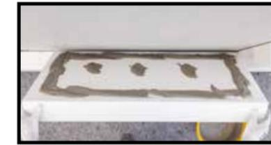
Installation of isolating panels with a notched trowel in a vertical direction
