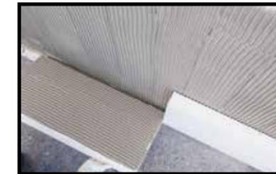
Installation of insulation panels with double buttering
