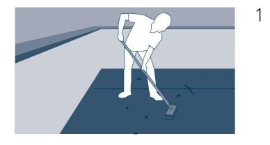
The installation on the plastic supports must only been done on perfectly waterproof substrates. Before proceeding with the installation clean the substrate thoroughly.
